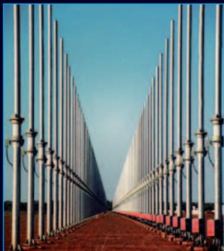
14. Jindalee Operational Radar Network (JORN), Laverton, Australien
